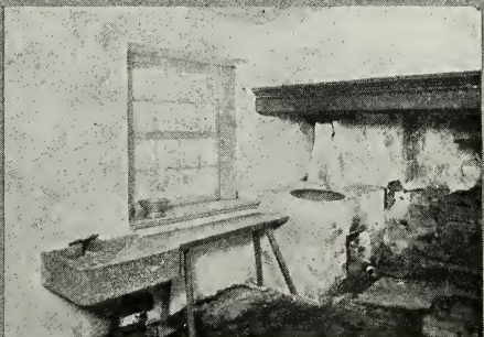
Saal kitchen, sink and drain pipe
