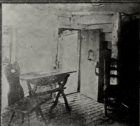
Sister House, or Saron. First floor Kitchen.
